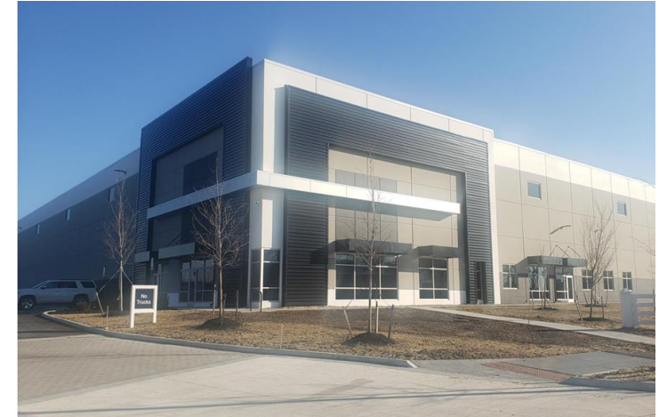
TriMas Packaging New Albany, Ohio, Facility Progress
